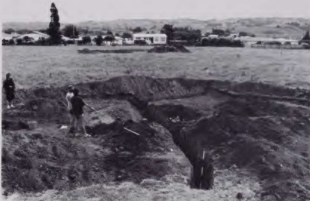
Fig. 18. Area IV, view to the north–west from outside the redoubt, across the defensive ditch to the pebble path into the bastion (at right of the two figures). The Area III excavation can be seen in the background.
